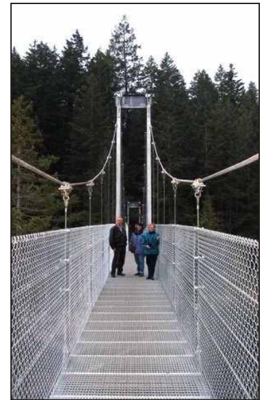
Regional District of Nanaimo Parks pedestrian bridge over the Top River near Parksville. Not on the TCT, but an example of what is happening on the Island. Photo by Jeannette Klein.
