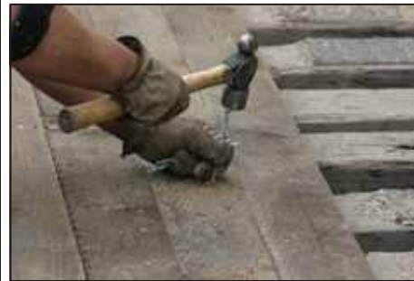
Laying down a new deck on Trestle 12. Murphy Shewchuk photo.
